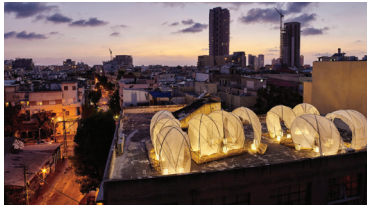
The mobile emergency response, Tel Aviv - Israel, 2019 The design was developed by the studio through 1:1 prototypes in a period of over a year. Photo: Dan Perez
